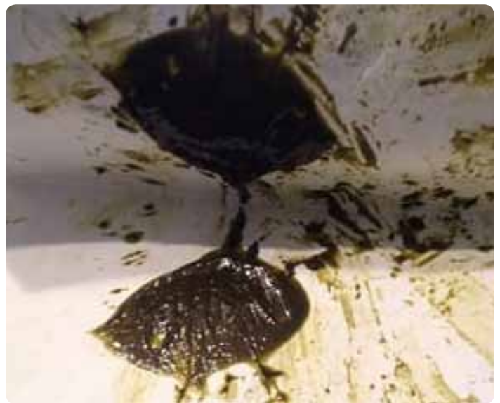
Tunnel Trimmer Extract
